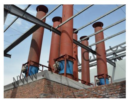
Smoke-releasing fan is installed at the above of firing zone in the kiln for discharging the smoke in the firing zone.
